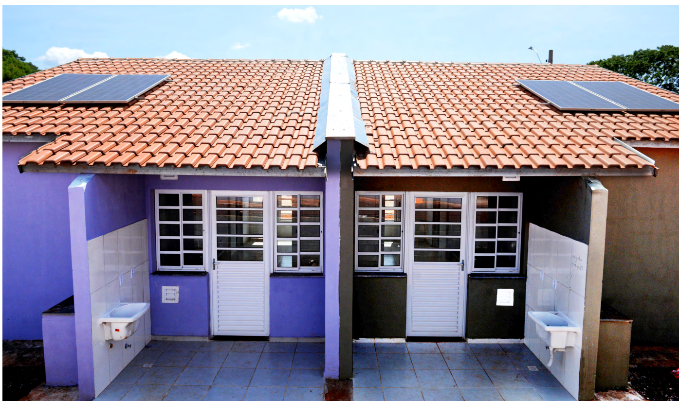
Photovoltaic energy device at the Aguai G development.
