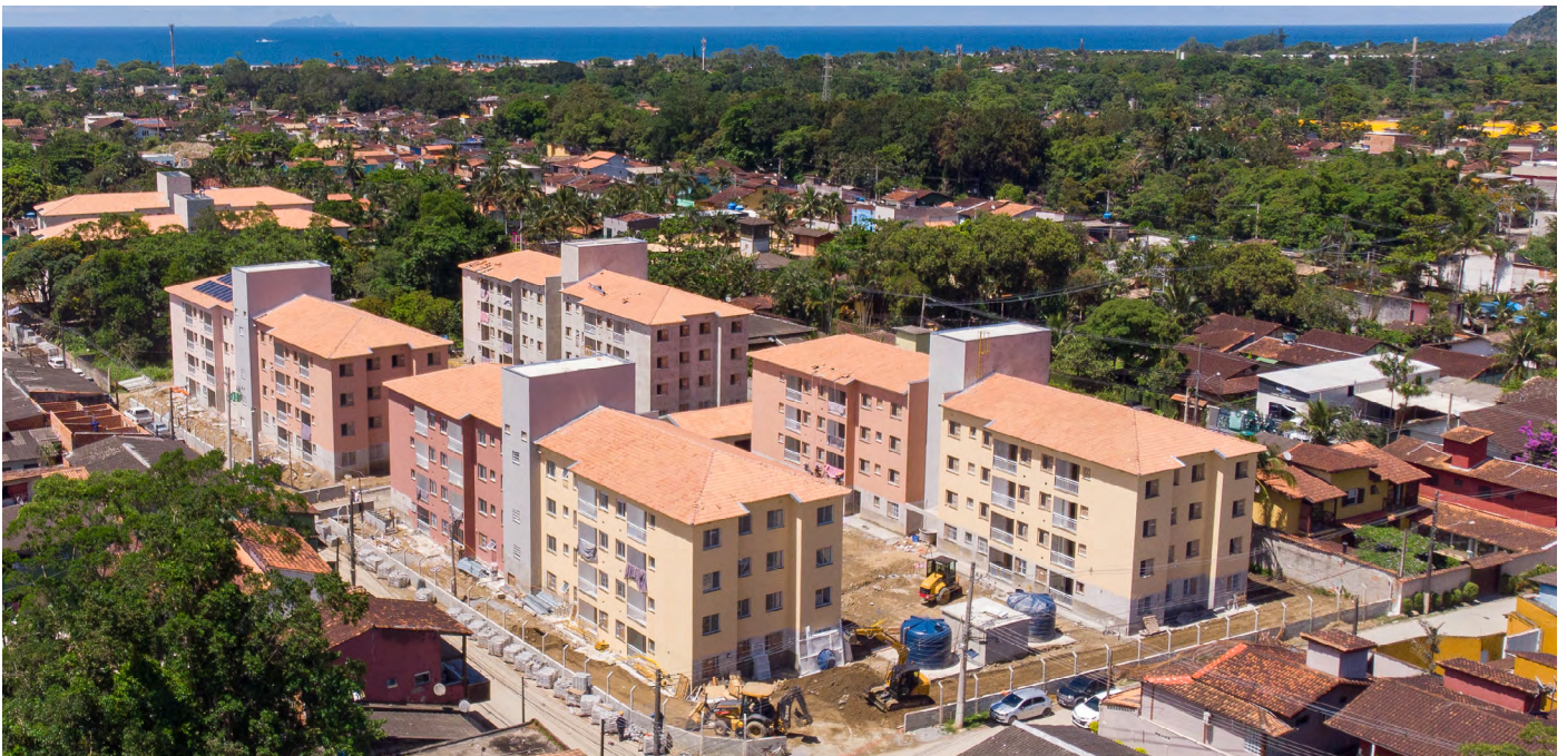
Construction work on the housing development in Maresias.
