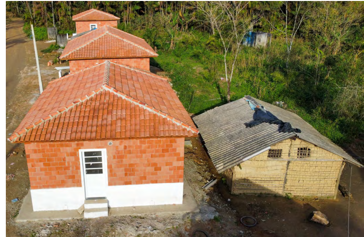
Indigenous Housing: original indigenous house and CDHU Bertioga E housing unit.
